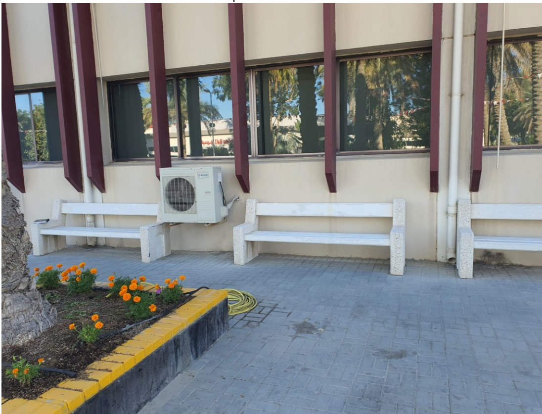
Figure 7. picture of building 28 taken in 2023 showcasing the difference in the colour of the louvres in Figure 6
