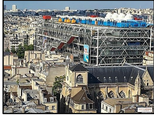
Fig. 03 : The Pompidou center in old Paris
