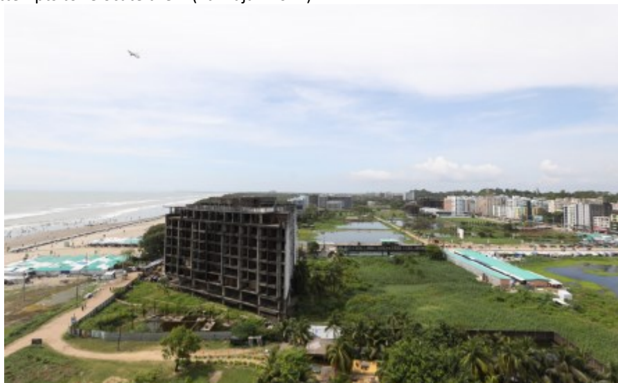
Figure 4: Unplanned hotels and motels are present on the prohibited area despite the fact that development is prohibited within 300 meters of the Cox's Bazar sea beach. Photo: Mohammad Minhaj Uddin (Faruque, 2021)
