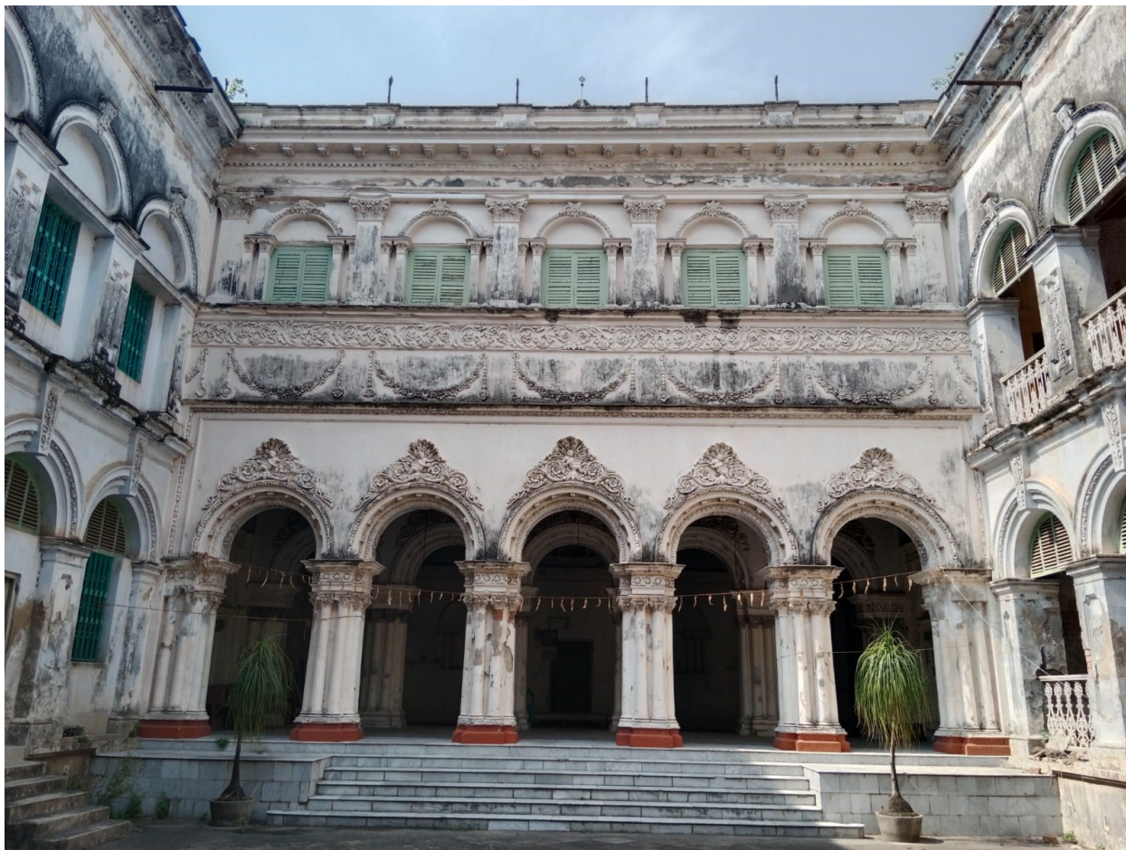
Figure 4. Sawoo Mansion showing Thakurdalan, stucco work on lunette, and insinuated wall above
