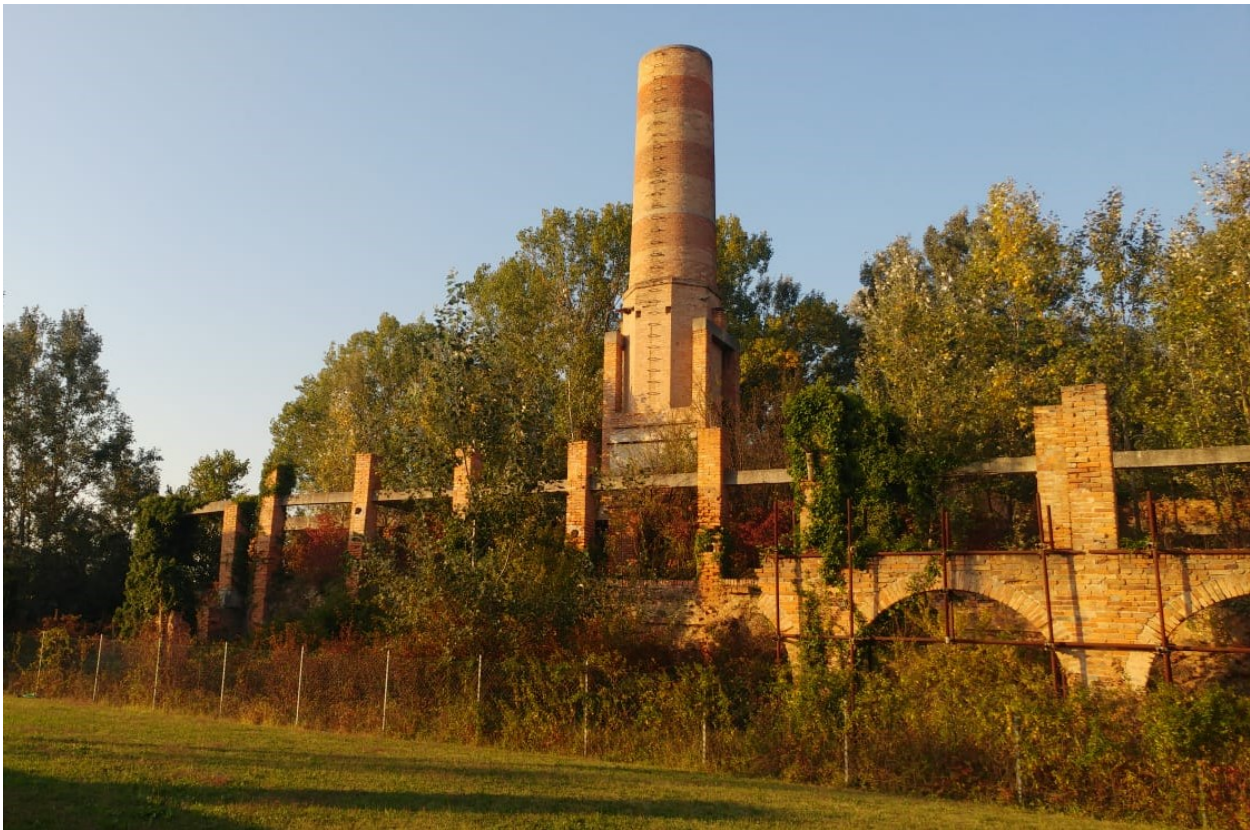
Figure 1. The ruins of the Morandi furnace covered by vegetation, seen from the south. Current state.
