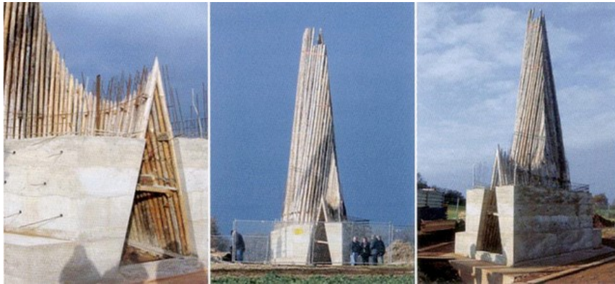
Figure 7. Construction of the sacral void, Bruder Klaus Field Chapel, architect Peter Zumthora source : https://de-architects.com/Feldkapelle-fur-den-heiligen-Bruder-Klaus-03-Bruder-Klaus-Field
