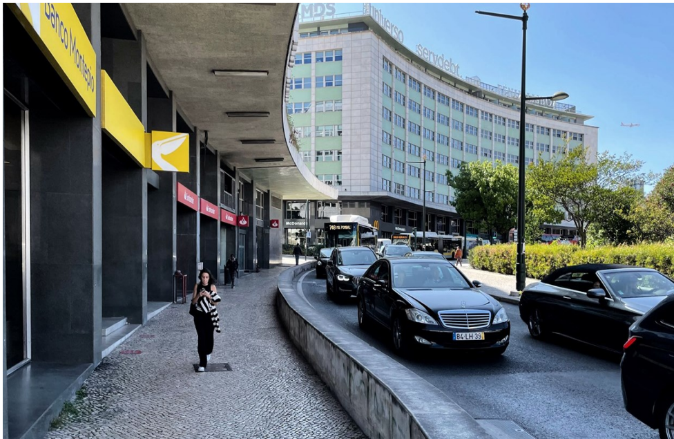
Figure 6. Loggia with cantilevered structure.
