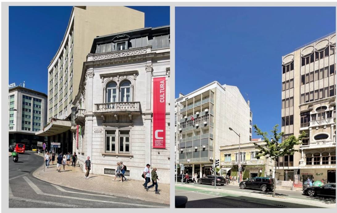
Figure 5. Introduction of a loggia in urban rehabilitation: roof protruding from the façade versus building plot.
