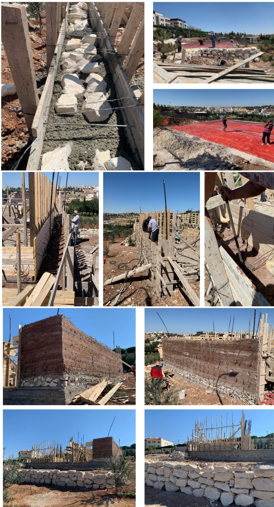
Figure 3. The construction process of the experimental rammed earth building (Authors).
