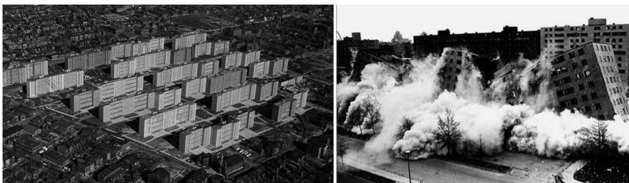
Figure 6. (left) Overall view of Pruitt-Igoe, public housing project constructed in St. Louis in the 1960s. (Newman,
