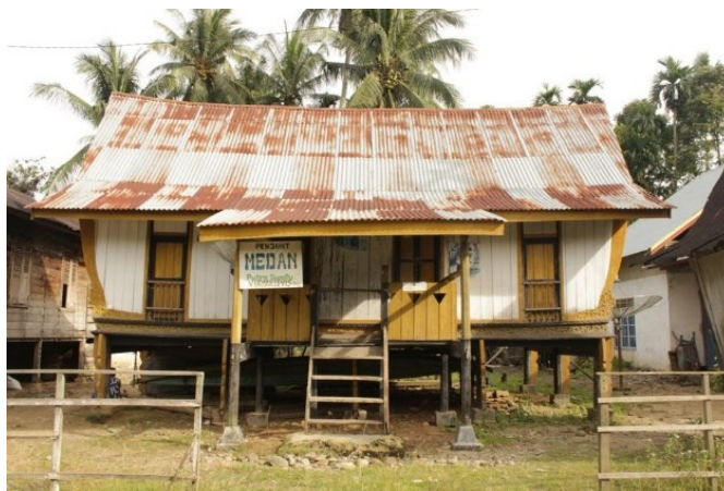
Figure 2. Malay house Rokan IV Koto
