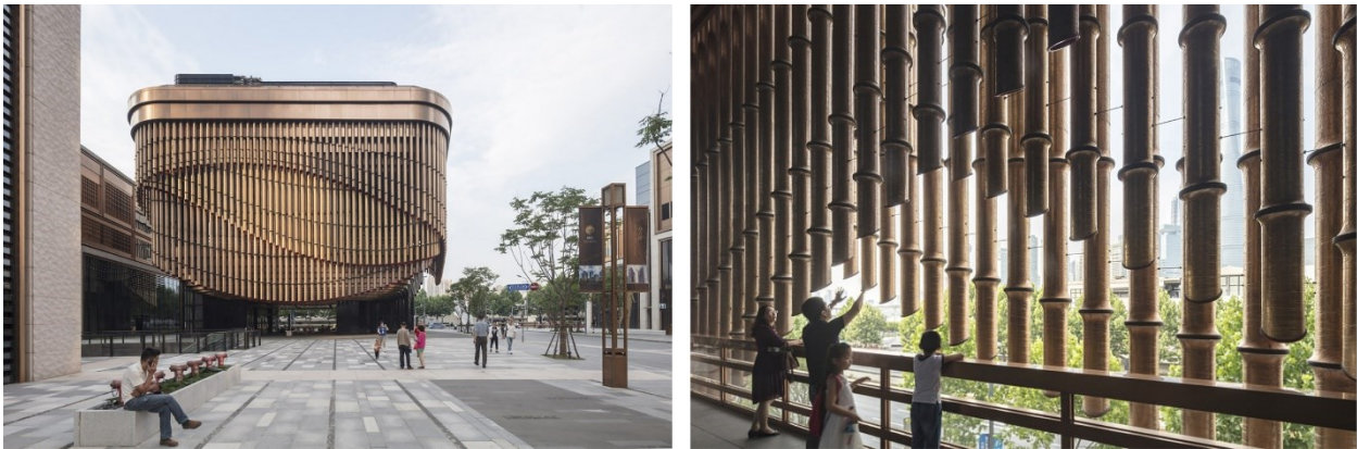
Figure 6. Bund Finance Centre (URL-5, 2021)
