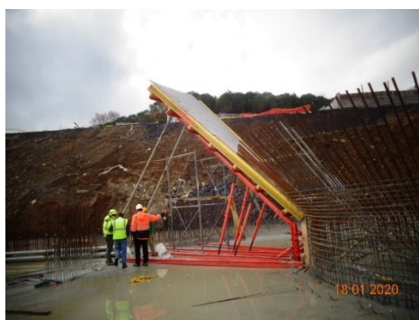
Figure 2. Installation of the formwork.
