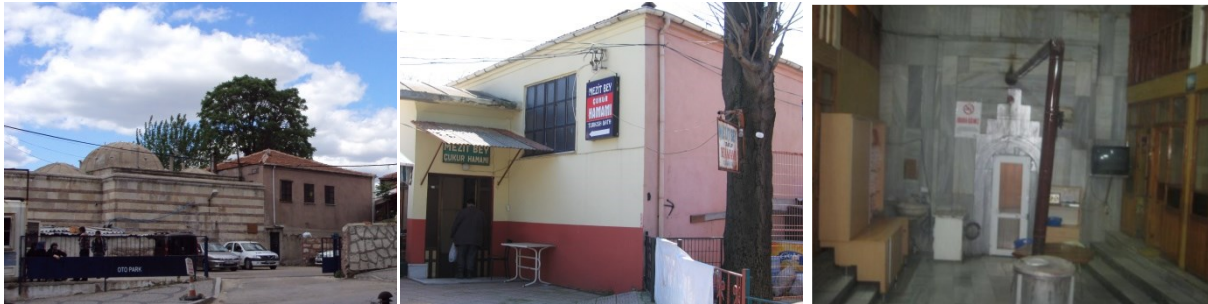
Figure 6. Northwest Wall of Mezitbey Bath on the Left (18.05.2010), Entrance of the Bath in the Middle (18.05.2010), Bath's Changing Room on the Right (Aşut, 2012).
