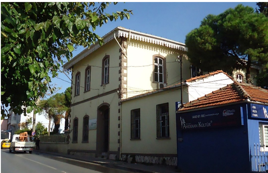
Figure 2. Front elevation of the mansion.
