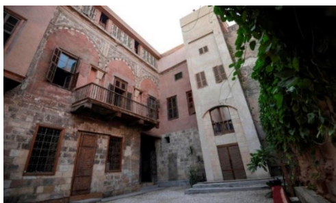
Figure 3. An Online image of "The Court of Bayt Yakan after restoration" ( https://www.thenews.com.pk/latest/390477-egypt-struggles-to-restore-cairos-historic-heart ).
