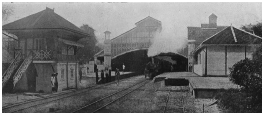
Figure 9. The old Kuala Lumpur Station that used one-sided having two platforms station plan type (Basri, 1985).
