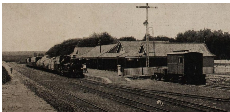
Figure 6. 1900 photographed of the one-sided station plan type of Newcastle Railway Station shows only one active platform for passengers used.
