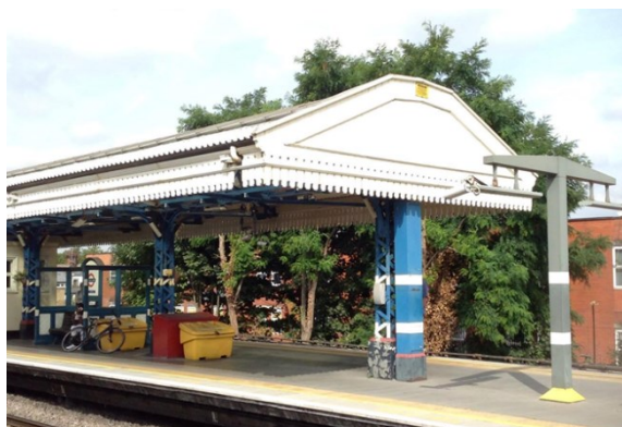
Figure 15. Turnham Green stations' train-sheds with steel column and timber panels as coverings (Fieldwork, 2016).
