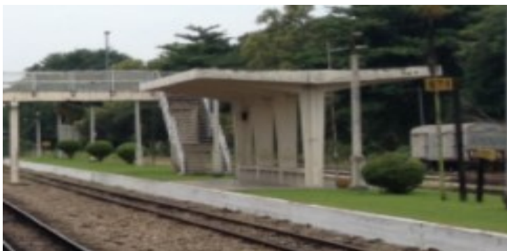
Figure 22. Kluang Station applied concrete butterfly shed at the island platform (Fieldwork, 2016).
