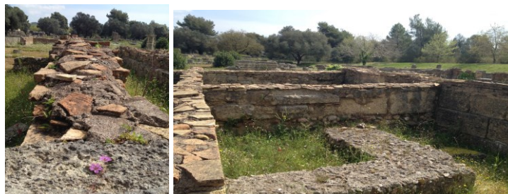
Figure 6. Sample for brick capping in Olympia/Greece (by author).
