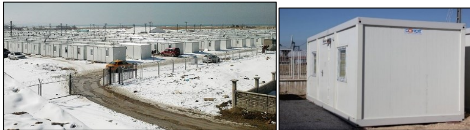
Figure 7. Temporary settlements in winter condition, one unit temporary housing (URL 5)
