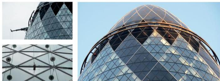
**Figure 38.** Rail and crane used for facade cleaning of Gherkin Tower(Boake,2014).
