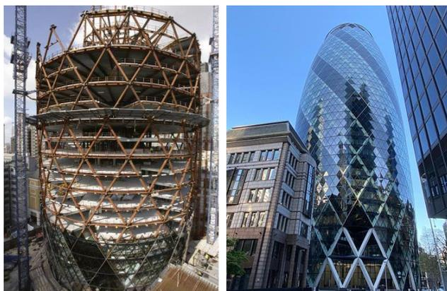
**Figure 23.** Construction aspect of the building (Munro, 2004).
