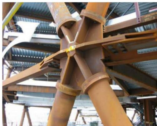
Figure 18. 3-story diagrid module and a triangular element sample(Asadi and Adali,2017)
