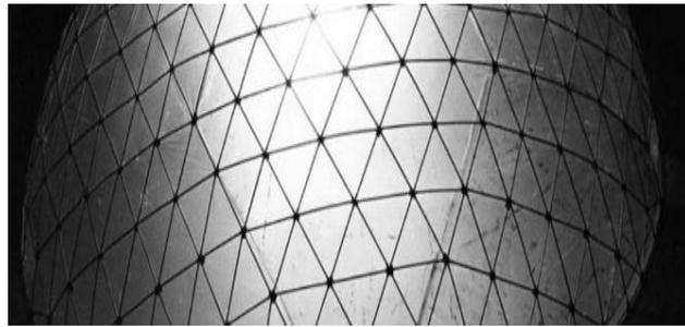
**Figure 9.** Division of a sphere by triangles (Baytin,2010).
