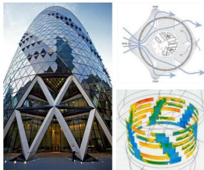
Figure 42. Ventilation system of Gherkin Tower(Shen,2009)
