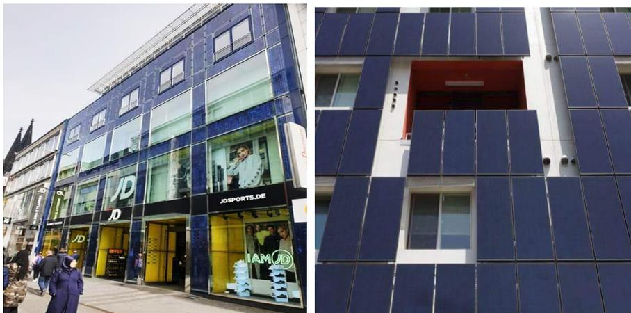
**Figure 3** install cells from the front facade building source developed by author
