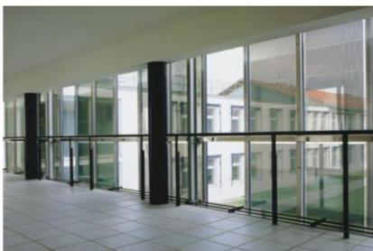
**Figure 10.** bipv installation , semi-transparent facad on thin film technology ( schott , 2018)
