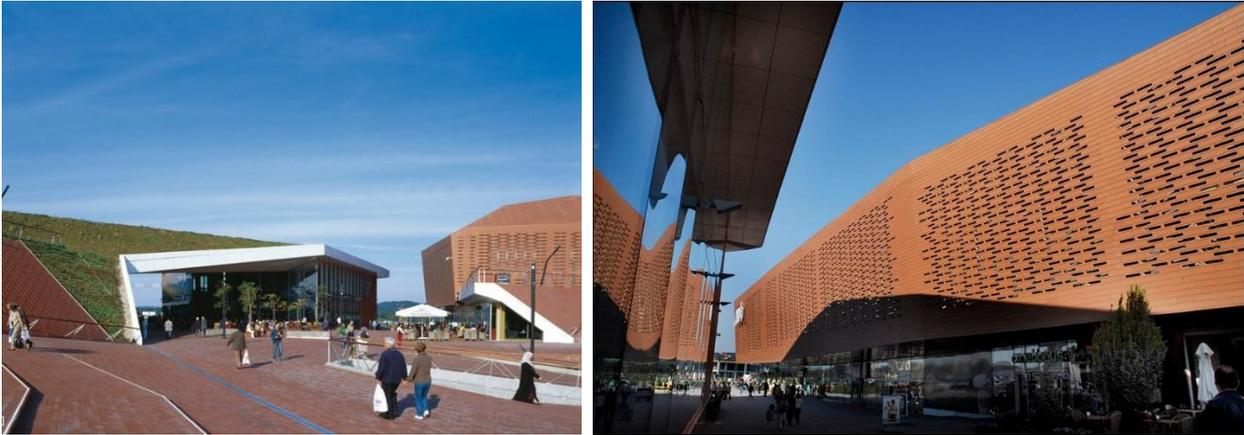
Figure 20,21. Earth colored façade and floor materials and green roof.
