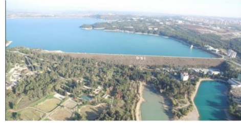
2: DSİ Dam Bridge
