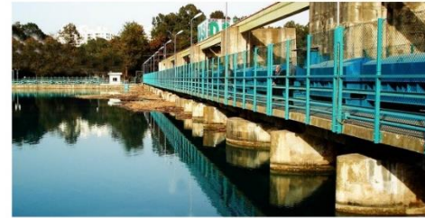
4: Seyhan Dam(DSİ) Bridge
