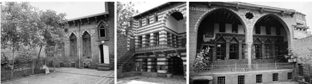
Figure 4: From left to right; courtyard, iwan and staircase patio examples (Bekleyen, Dalkılıç, 2011) Windows have large reveal depths because they are placed at the back of the window recesses. This helps to increase shading effect of the rooms and lower the greenhouse effect (Sözen & Gedik).
