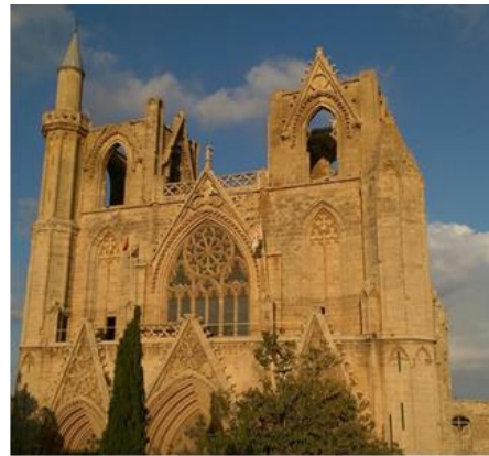
Figure 2. West Façade of the Cathedral of St. Nicholas (Babazadeh Asbagh, 2019).
