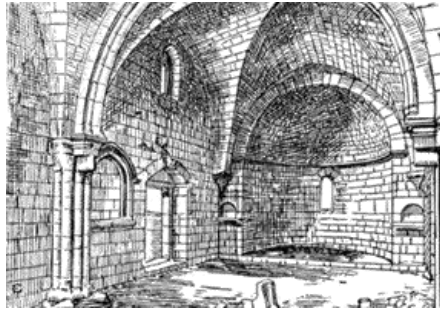
Figure 23. Interior View of Jacobean Church (Enlart, 1987, p. 301).
