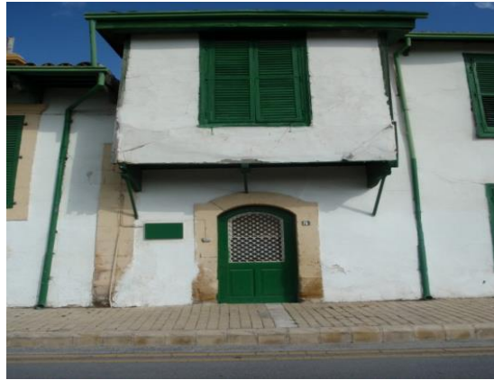
Figure 3.4 Arabahmet Neighbourhood Bay Window Façade. Source: Author
