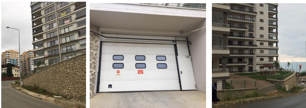
Figure 6. Fieldwork images of Seyri Şehir Houses
