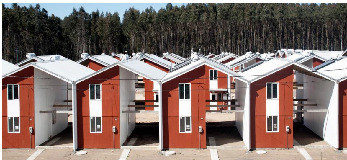
Figure 2. Villa Verde Housing by ELEMENTAL (Archdaily.com).
