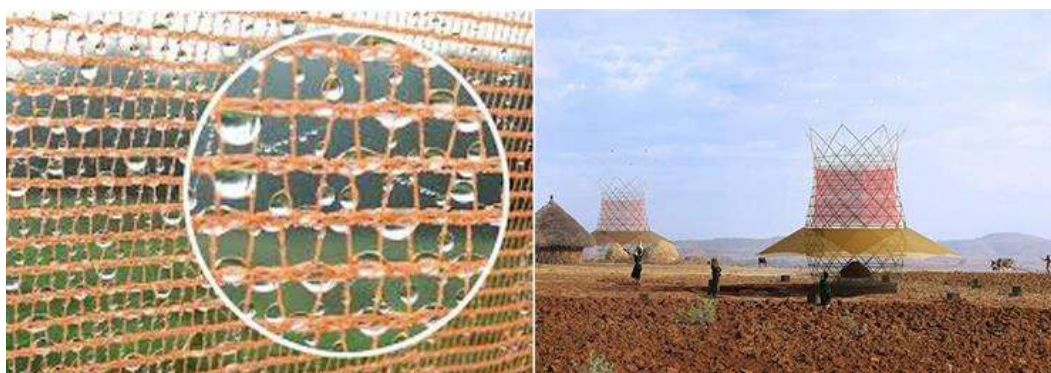
Figure 4. (A Warka water tower Bamboo Tower That Produces Water from Air) (URL 4)
