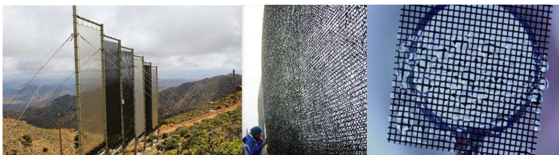
Figure 2. Collecting desalinated water through fog (URL2)
