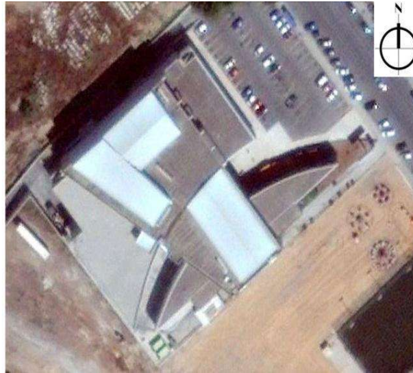
Fig 7. Aerial View of Lemar Shopping Mall (Image Courtesy of Google Map, 2017)
