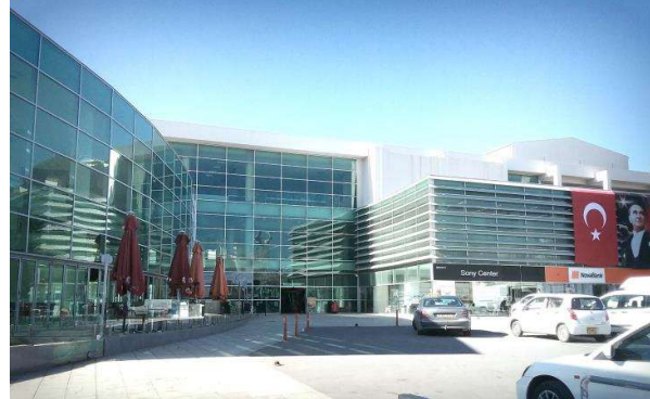
Fig 8. Main Approach to Lemar Shopping Mall (North-Eastern Elevation) Showing Shaded Entrance to Mall. (Chinweokwu and Alibaba's Archive, 2017)
