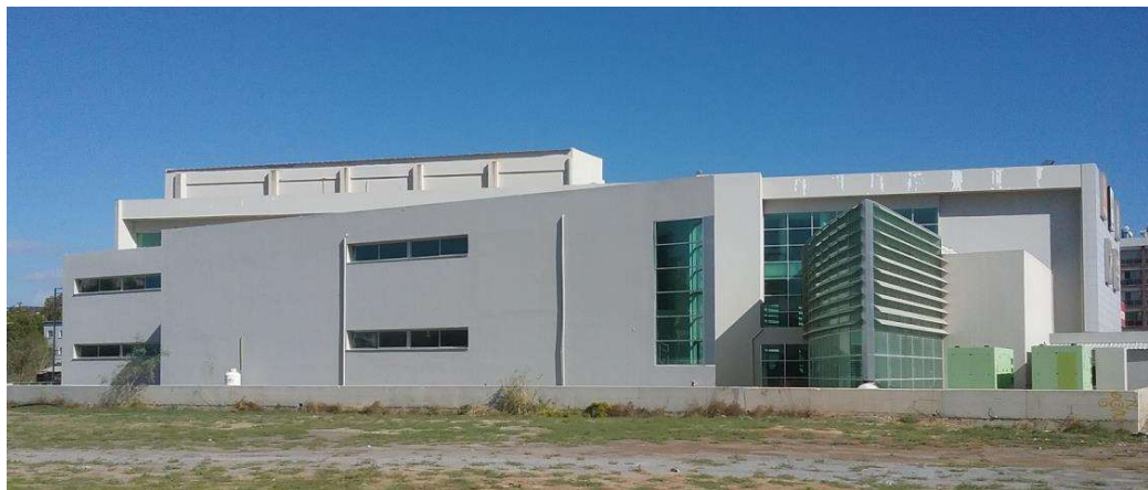
Fig 11. South Western Elevation Showing Partial Recessing and Use of Shading Louvers (Chinweokwu and Alibaba’s Archive, 2017)
