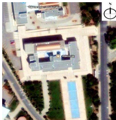
Fig 1. Aerial View of Emu Rectorate Office Building (Image Courtesy of Google Maps, 2017)
