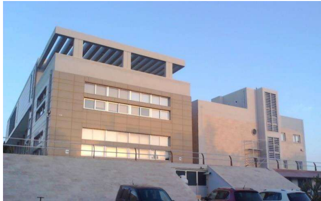
Fig 4. Concrete Pergola over Terrace - Western Facade (Chinweokwu and Alibaba's Archive, 2017)
