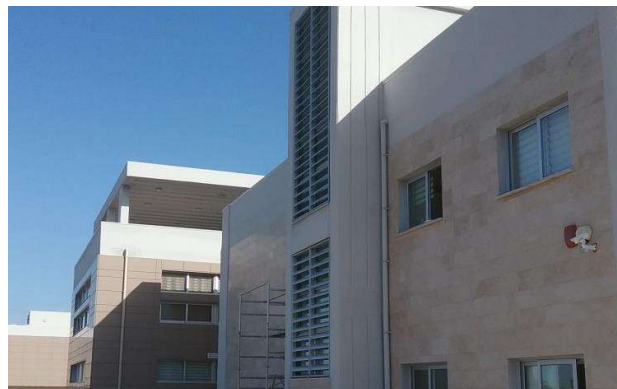
Fig 6. Selective Shading of Windows at Emu Admin Building - West Facade (Chinweokwu and Alibaba's Archive, 2017)
