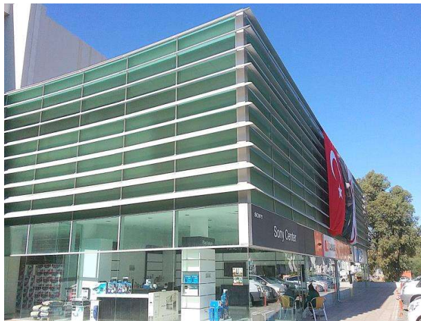
Fig 10. Continuous Horizontal Aluminium Fins Employed on Upper Facade of Lemar Building (Chinweokwu and Alibaba's Archive, 2017)
