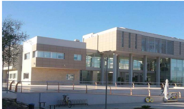
Fig 2. Showing Sunrise on Eastern Elevation and Suspended Floor on Northern Elevation (Chinweokwu and Alibaba's Archive, 2017)
