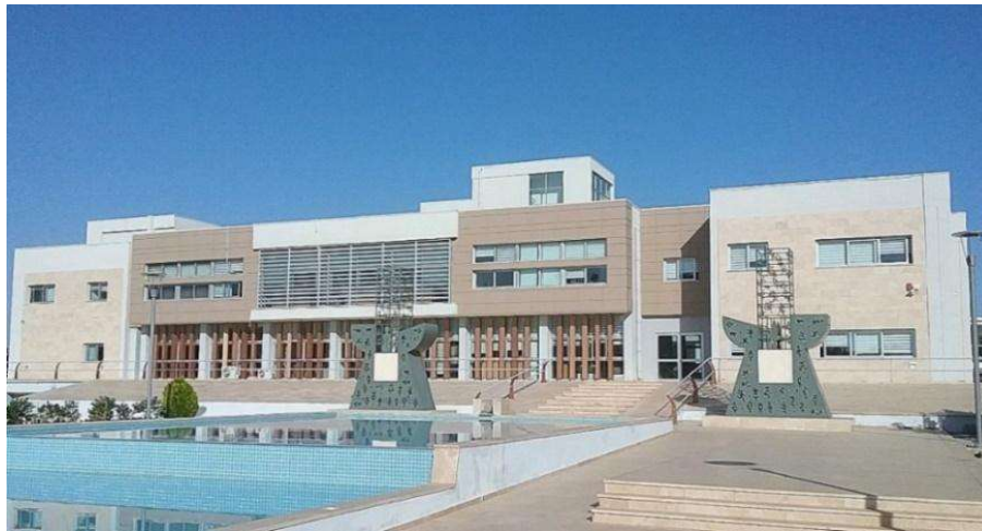
Fig 5. Showing Facade of Emu Rectorate Office - South Facade (Chinweokwu and Alibaba's Archive, 2017)
