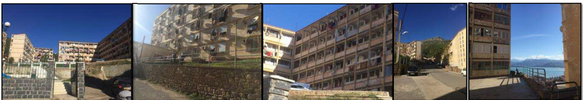
Figure 10 . View on a type of collective housing (Amimoun)
