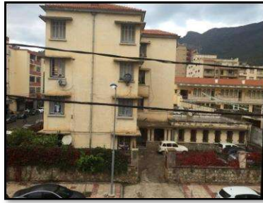
Figure 7. View on a type of collective housing (Lekhmis)
