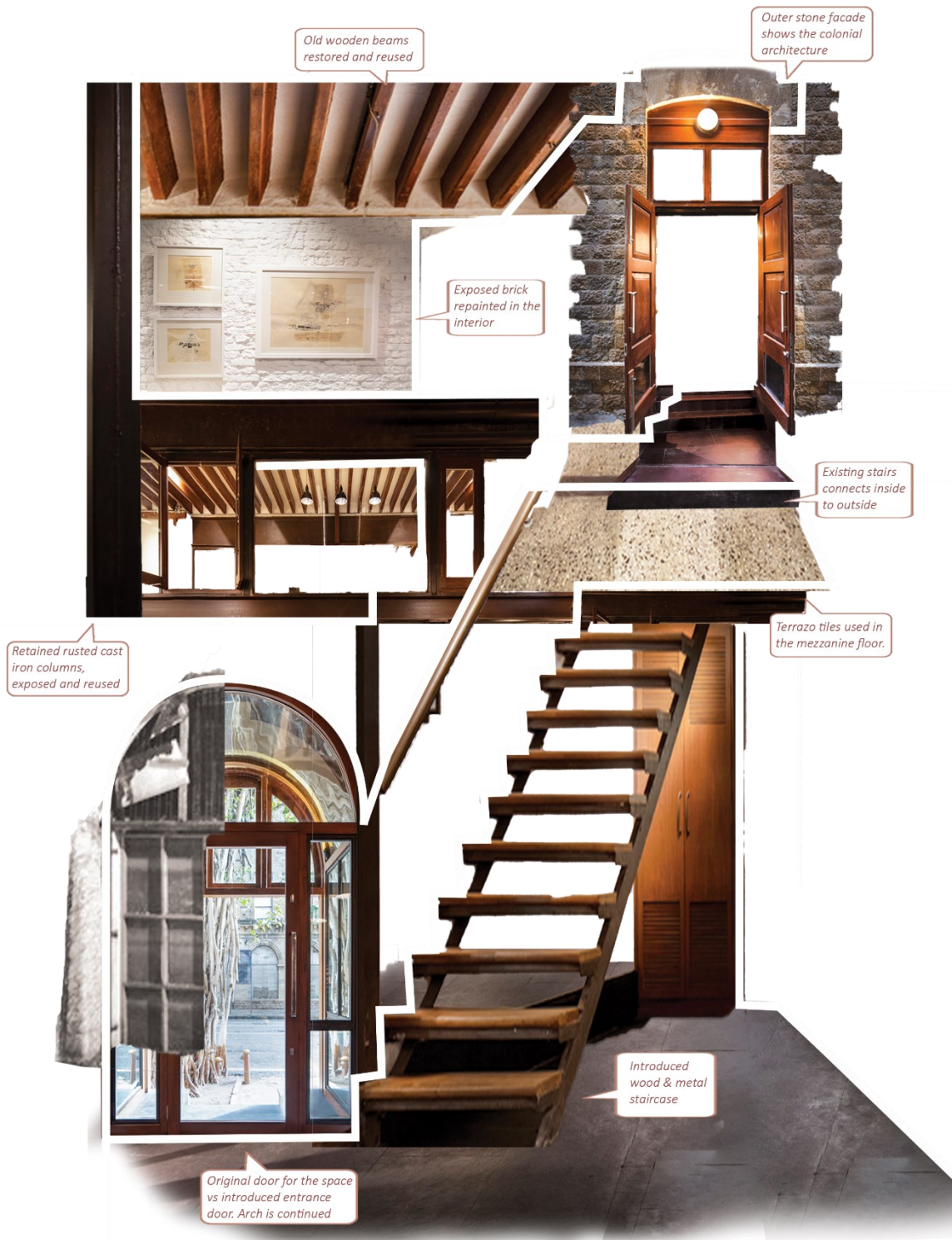
Figure 4. Collage showing the interplay of retained and new material in the furniture studio Tianu, Mumbai
