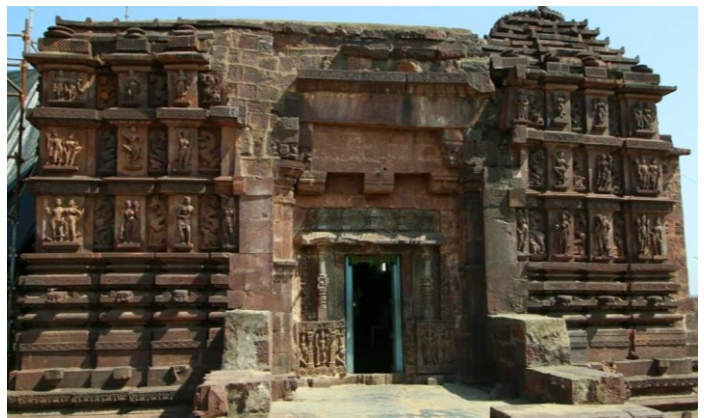
Figure 3: Current restoration of the temple.
