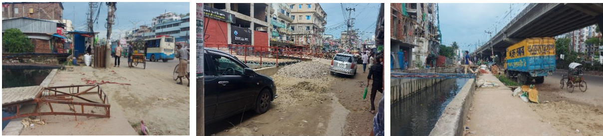
Figure 4: Existing condition of the study area
