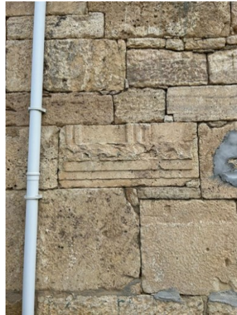
Figure 3. A cornice detail.
