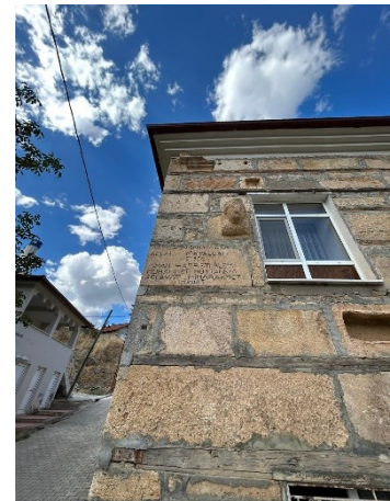
Figure 7. Usege details of ancient materials on the mosque façade.
