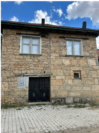
Figure 5. Ancient material usage on facades.
