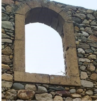
Figure 6. Minasin Mill window detail (Prepared by the authors).
