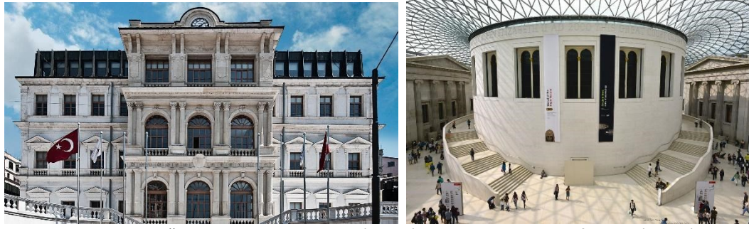
Figure 1. Beyoğlu Municipality Building (URL 1), British Museum roof annex (URL 2).
