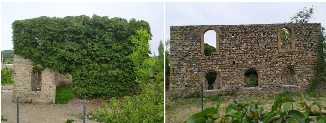
Figure 4. Minasin Mill north and south facades (Prepared by the authors).
