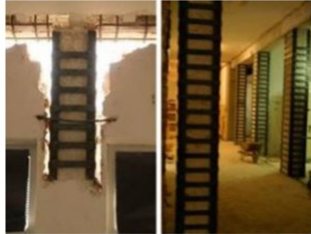
Figure 1. Retrofitting of RC frames with steel caging [21]
