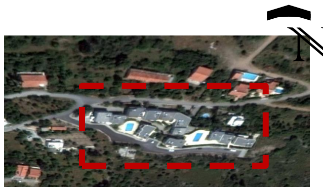
Figure9: New construction in Karmi village
