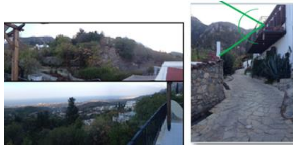
Figure 16, 17 and 18: View of Old construction building in Karmi village
