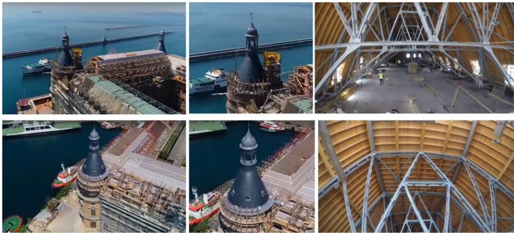
Figure 19. Haydarpasha Railhead Restoration Works after 2010 Fire
