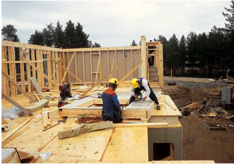
Figure 4. Typical platform-frame construction in Oulu, Finland in 1996.
