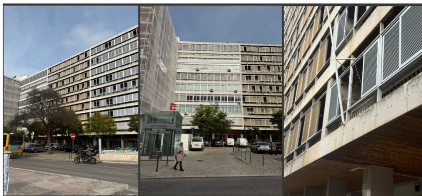
Figure 3. Private Loggias (Alvalade Square in Lisbon).
