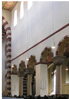
Figure 7. Piers and columns.
