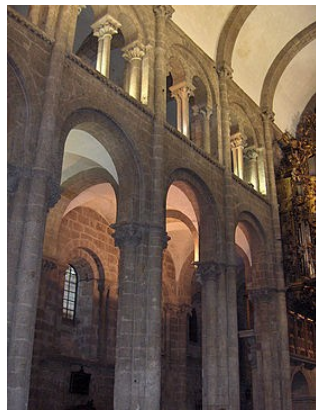
Figure 6. Piers and columns.
