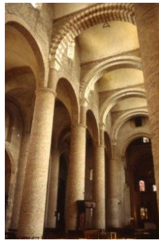
Figure 10. Barrel vault.
