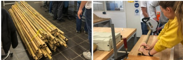
Figure 4: Moving the bamboos to the workshop and cutting. Own Source, Abanoz, B., 2025.
