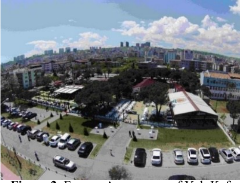
Figure 2. Former Appearance of Yalı Kafe.
