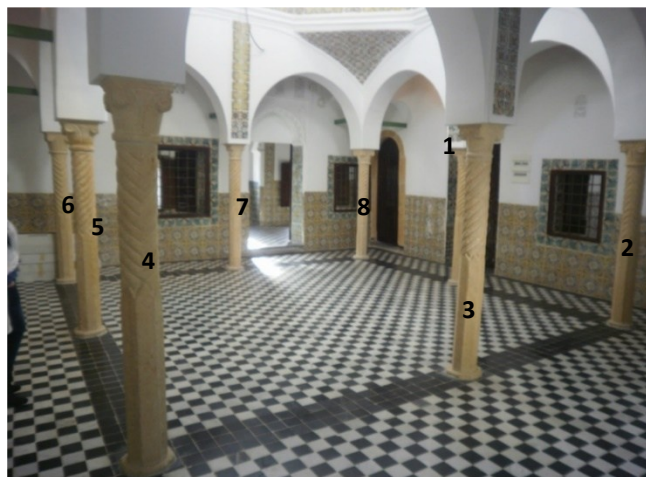
Figure 1. The eight columns of the patio intended for restoration (Bardo Museum, 2012).
