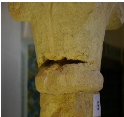
Figure 7. The loss of stone at the level of columns 5, 6 and 7.
