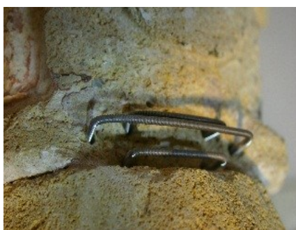
Figure 8. Insertion of stainless steel cores (columns 1-5 and 7).
