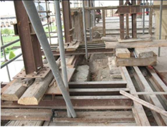
Using wooden crossbars under column bases.
