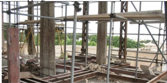
Wrapping with iron beams on the porch floor.
