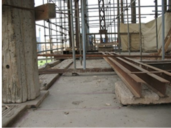
Scaffolding and Floor wrapping.
