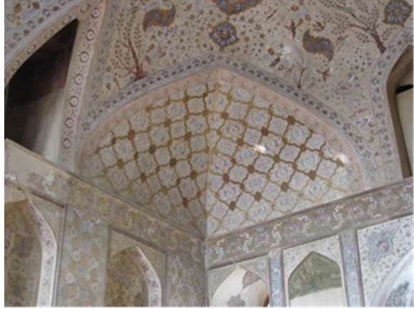
Corner construction for arch construction.
