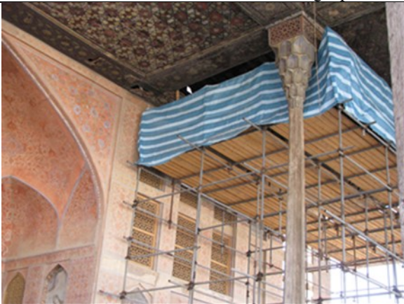
Scaffolding for roof repair and covering the workshop area of Aalighapu.
