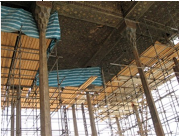
Installing scaffolding for roof and column repairs.
