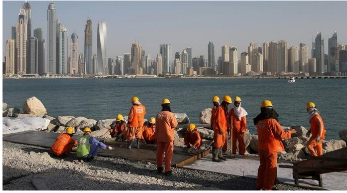
Figure 6. Construction site and migrant workers in Doha.
