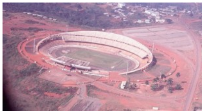
Figure 4.5: Ahmadou Ahidjo Stadium Original Structure (Mangaleu Toukam, 2023)
