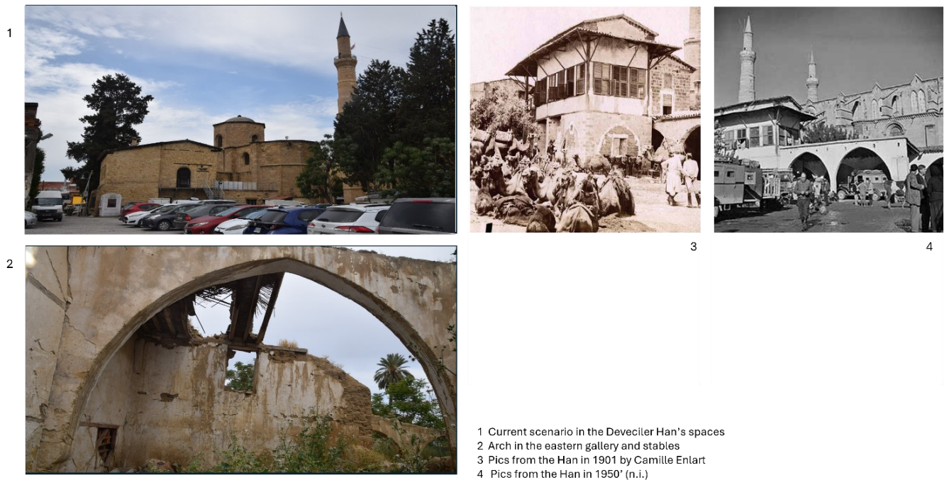
Figure 7. Current state of Deveciler han.
