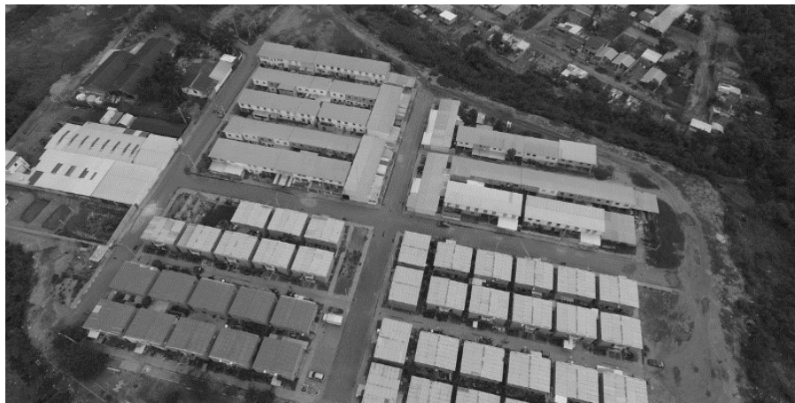
Figure 1. A post-disaster settlement from Ecuador (University of Leeds, n.d.).
