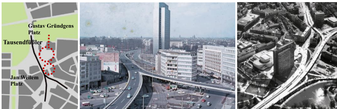
Figure 3. Aerial views of the Tausendfüßler elevated road between the Hofgarten and Jan-Wellem-Platz before its demolition, and Jan-Wellem-Platz (a. Stöfer (2006), b. Linksfraktion Düsseldorf (2008), c. HPP Architekten (n.d.)).
